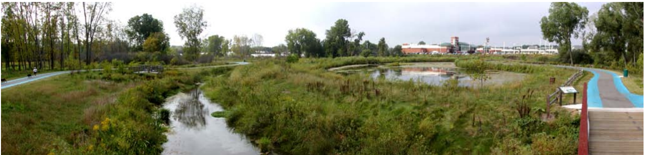
Figure 3. Panoramic view of the completed Regional Stormwater and Trailways Facility.
